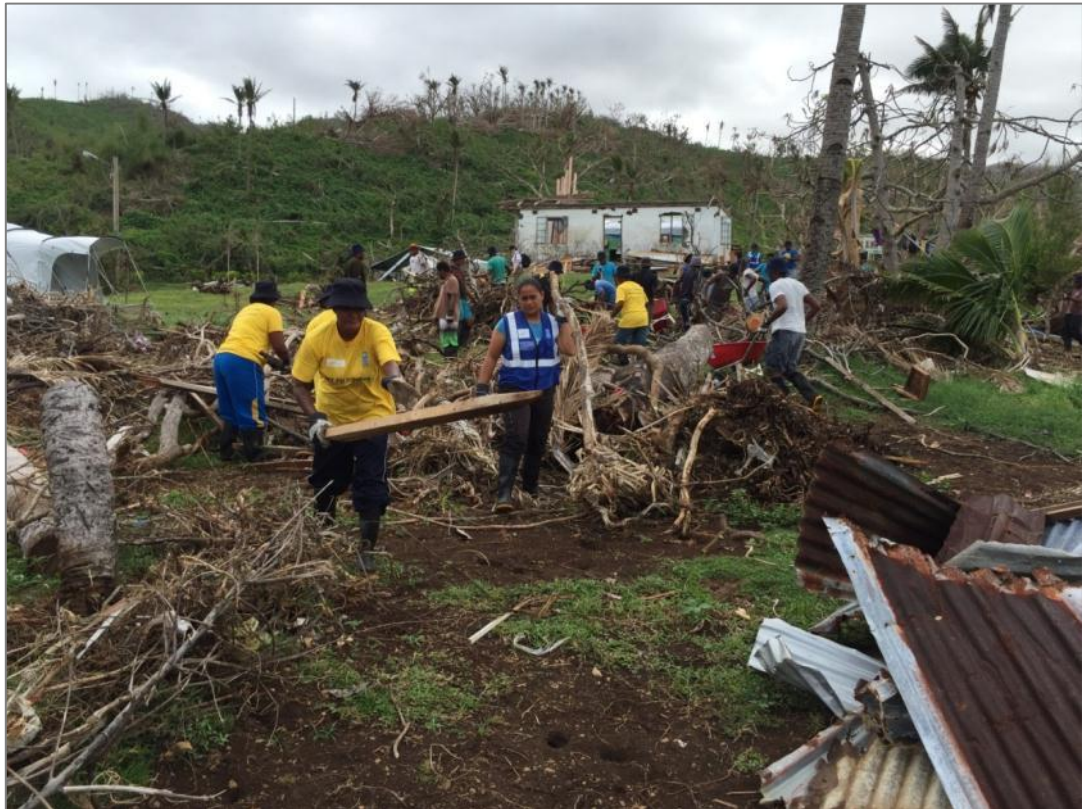
Figure 3 – Debris clearance in Koro Island – Namacu village (photo credit: Faisal Ridwan)
